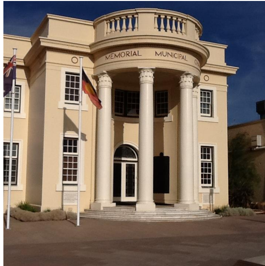
Kerang Memorial Municipal Chambers (Photo from AWM – Places of Pride – Trevor Linton)
